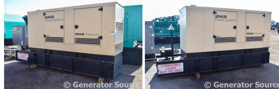
**Description:** Kohler 150 kW Diesel Generator Model #: 150REOZJF Serial #: SGM32BCZ5 Year 2014, 150 Hours, 277/480 Volt, 3 Phase, Sound Attenuated Enclosure
